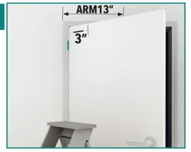
On the door measure 3" away from the hinges for Model 133 and 4" for Model 233, then create a mark. This is where the operator will need to be positioned. On the door jamb, measure 13" and create a mark, this is where the middle of your arm will need to be positioned. The bracket will need to be as flush as possible with the wall. Do not mount this bracket at an angle.
